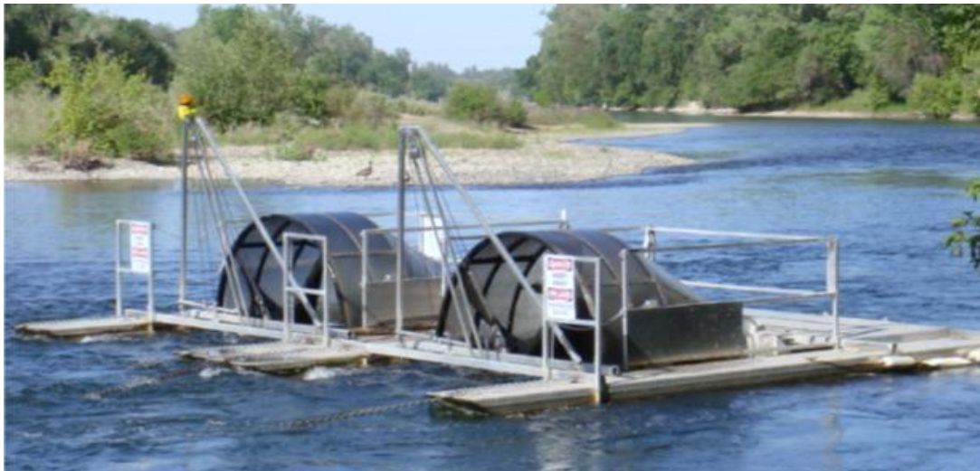
Figure 2: The two north channel 8 foot traps (8.1 and 8.2) on the lower American River just downstream of the Watt Avenue overcrossing.
